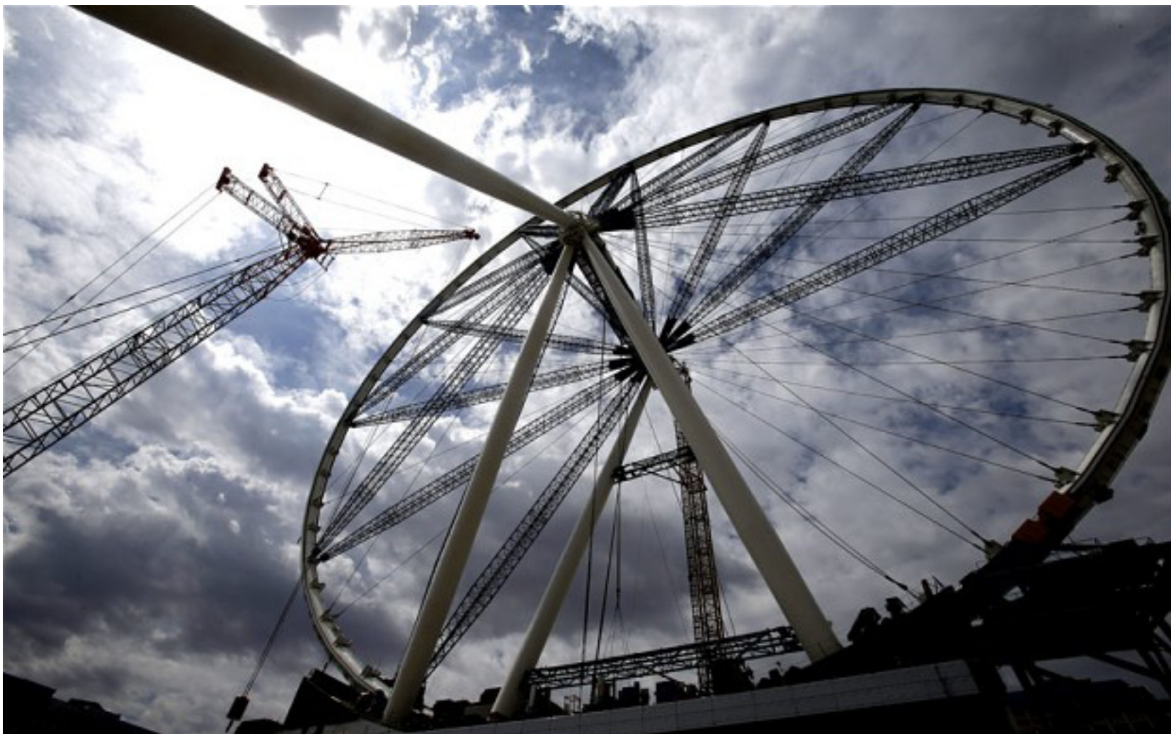
The final rim piece is added to the 55-story High Roller Ferris wheel under construction near the Las Vegas Strip. The ferris wheel will break the record for worlds largest when it opens in early 2015. | Photo credit: Isaac Brekken, AP Photo.
